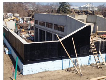
Elliot Construction moved upward from building residential basements. Photo: ELLIOT CONSTRUCTION
